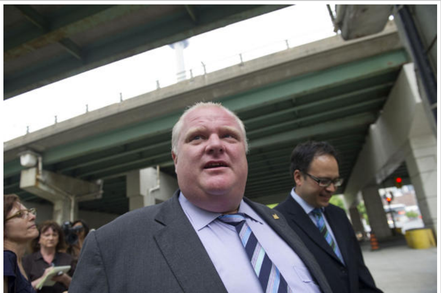
Mayor Rob Ford walks with Councillor Denzil Minnan-Wong (right) under the Gardiner Expressway as the two survey the work being done by crews to fix the falling debris on May 25, 2012.
