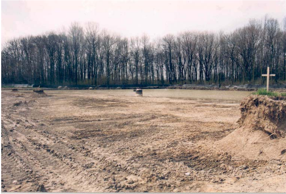
Figure 17 - Example of large scale removal of natural soil during site development
