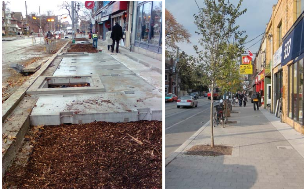
Figure 21 - Roncesvalles Boulevard during sidewalk reconstruction and after.
