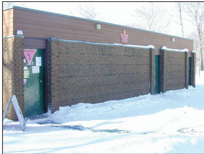
No windows in staff room, Kew Rink
