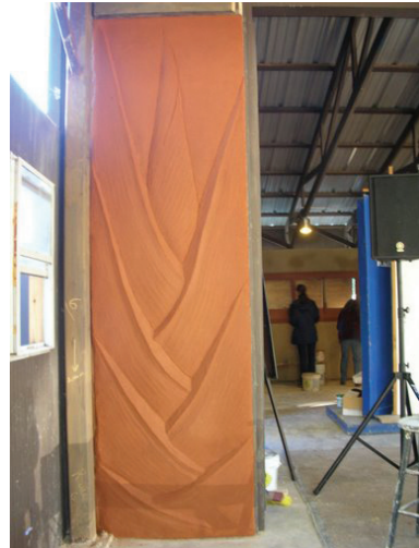
Earthen plastered wall in Texas
