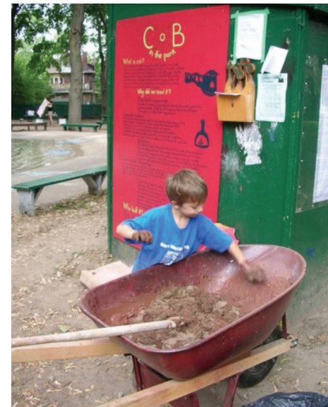
Mixing up dried clay for earthen plaster
