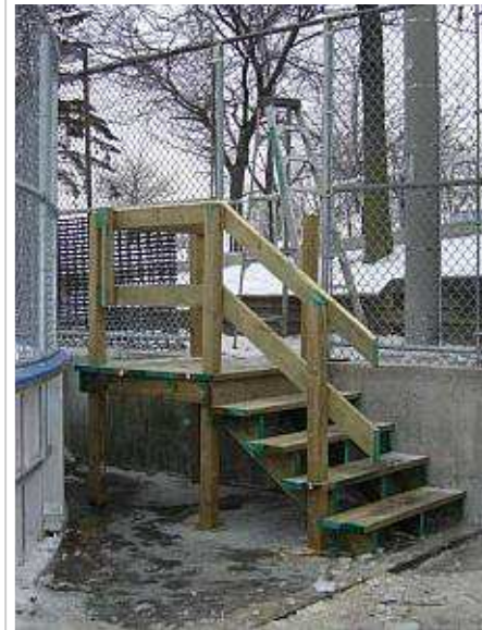
new rink access stairs
